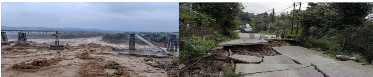
Chakki Bridge and roads in Dharamshala damaged during August 2023
