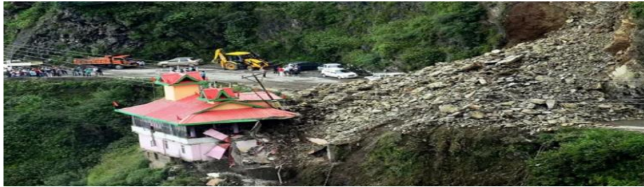
Landslide in Shiv Baori summer hill, Shimla
