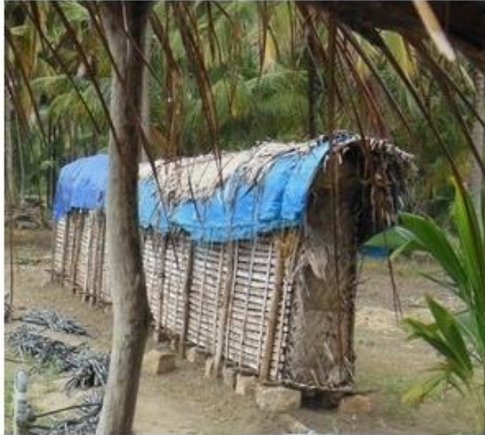
Onion storage structure i.e. Pattarai
