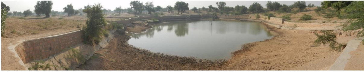
Fig-2. Improved Nadi with LDPE lining
